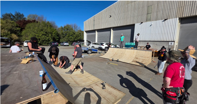
Surfacing one ramp face with coping already installed.
