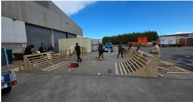
Multiple stations progressing in parallel.
