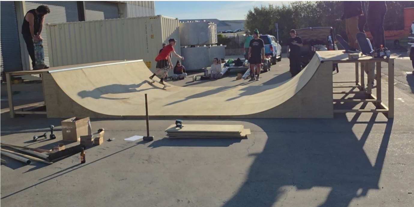
Completed ramp during the first build and test session, 26 September 2026.
