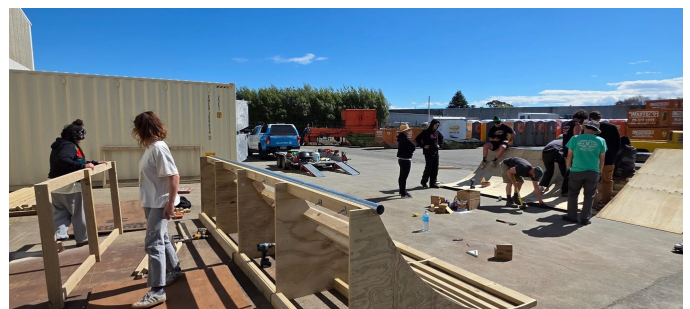
Platform-extension frames built alongside the ramp sections.
