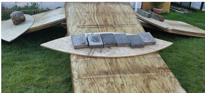
9 mm transition sheets wet and pre-bent before build day.
